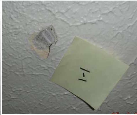
Sample 1-1, Texture/Plaster/Skim Coat, Kitchen
