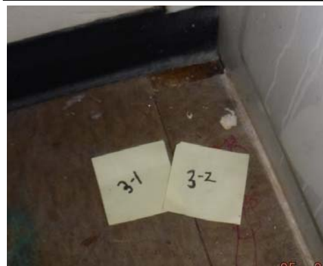
Samples 3-1, 3-2, 12" Floor Tile/Mastic, Bathroom
