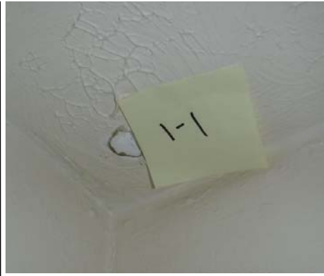
Sample 1-1. Texture/Drywall, Kitchen
