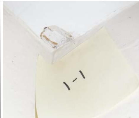
Sample 1-1, Drywall/Joint Compound, Kitchen
