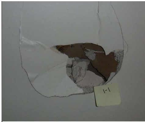
Sample 1-1, Plaster/Skim Coat, Dining Room
