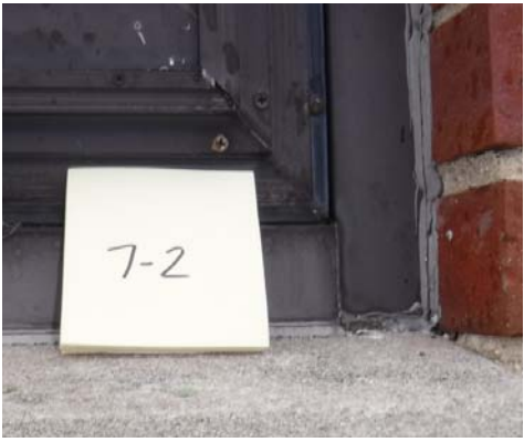
Sample 7-2, Window Caulk, Exterior
