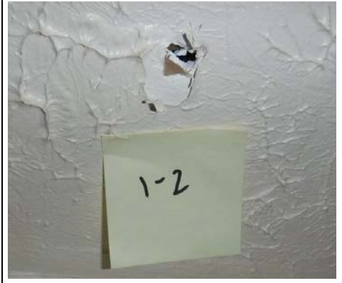
Sample 1-2, Texture/Drywall, Kitchen
