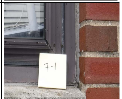
Sample 7-1, Window Caulk, Exterior
