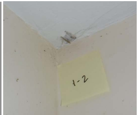
Sample 1-2, Drywall/Joint Compound, Kitchen
