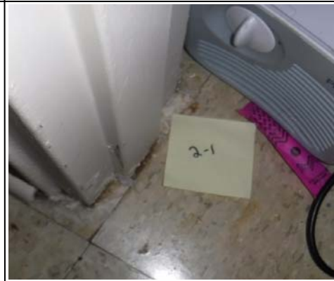
Sample 2-1, 12" Floor Tile/Adhesive, Hall Closet
