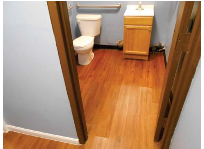
52. 1801 Attucks, community building restroom
