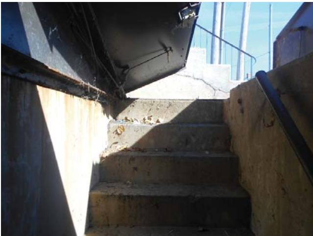
111. Typical basement stairs from entrance
