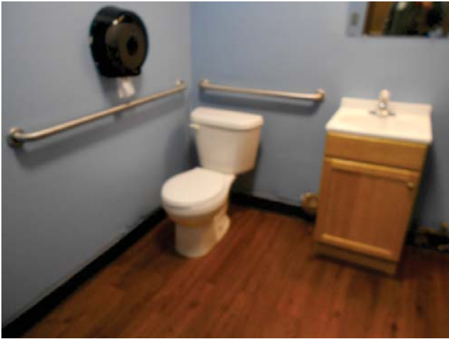
53. 1801 Attucks, community building restroom
