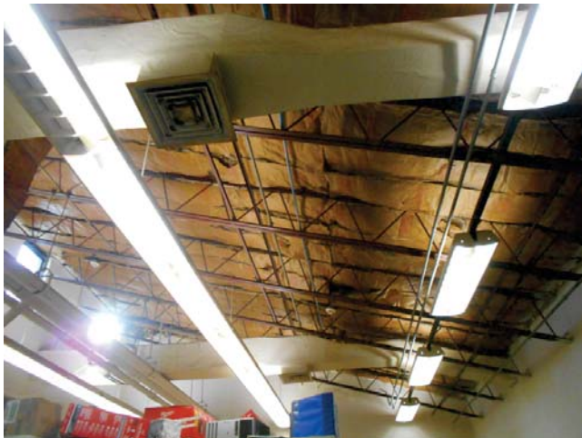
43. Leasing office maintenance offices ceiling
