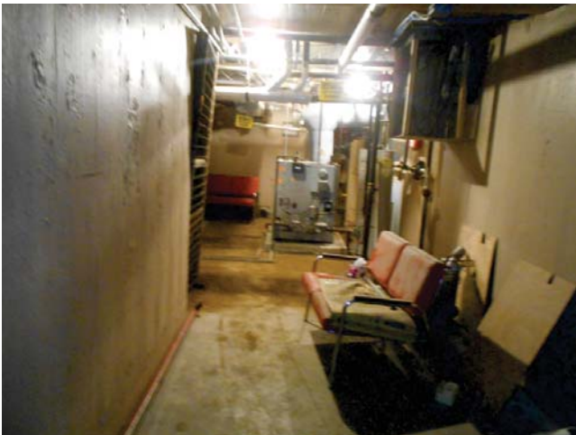
59. 900-914 Wilberforce Place, Task Force HQ, Mechanical Basement
