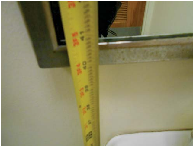
19. Leasing office public restroom, mirror height, 40"
