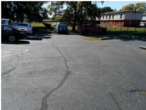
Leasing office asphalt parking lot
