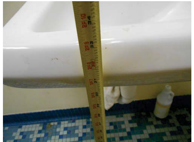
16. Leasing office public restroom, sink height, 34"
