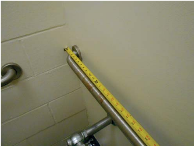
13. Leasing office public restroom, rear grab bar
