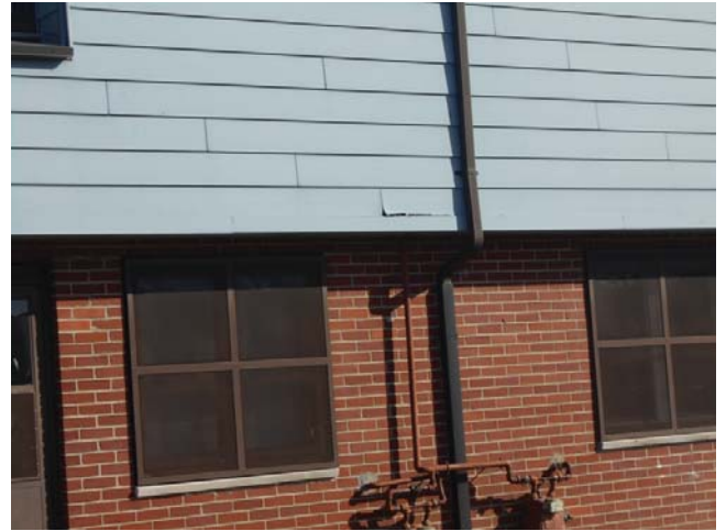
126. Typical section 502 building, older exterior siding
