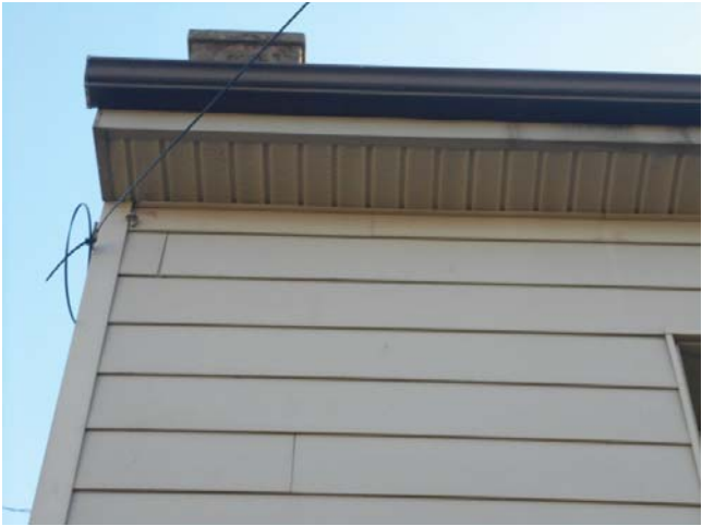
158. Typical soffit condition
