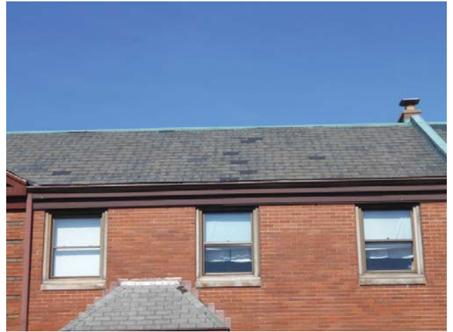
106. Typical slate tile roofing
