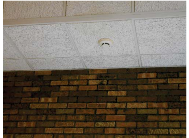
6. Leasing office entrance smoke detector
