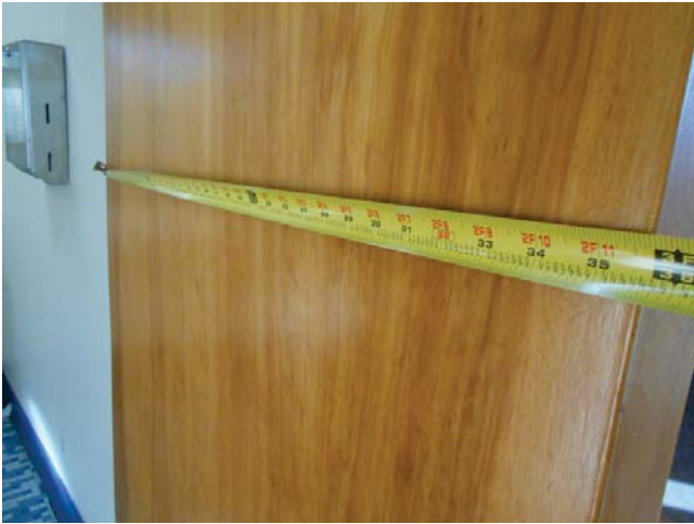
9. Leasing office public restroom door width, 36"
