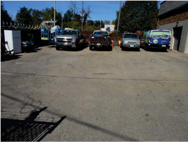
81. Leasing office asphalt parking lot
