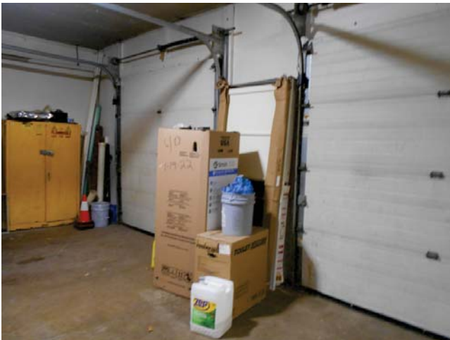
27. Leasing office maintenance garage
