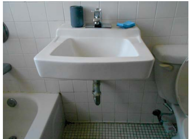
12. 818 Oldfield Avenue, 1bed/1bath, upstairs unit, vacant - Bathroom
