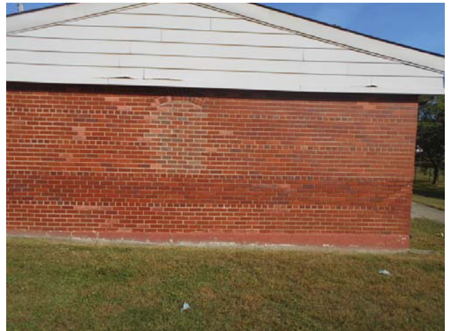
140. 86-96 Benning Place, Side facade
