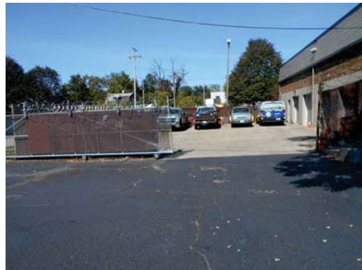
Leasing office asphalt parking lot
