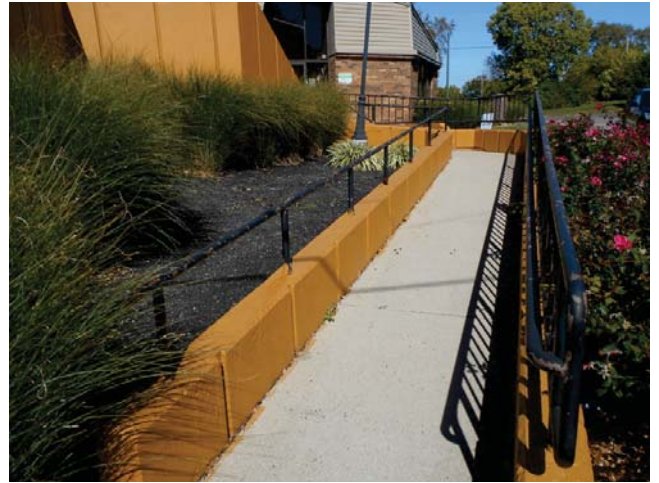
94. Leasing office main entrance
