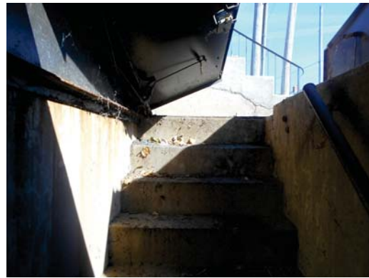
Typical basement stairs from entrance
