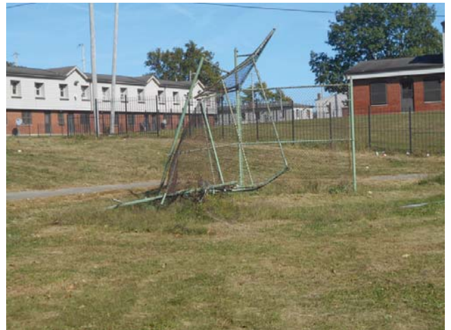
156. Damaged chain-link fencing in Gillespie Park
