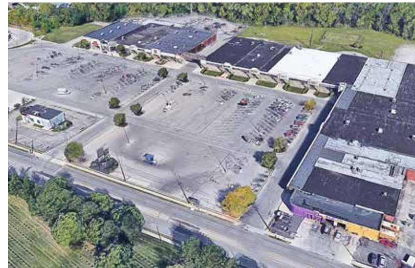
View of existing conditions looking northwest
