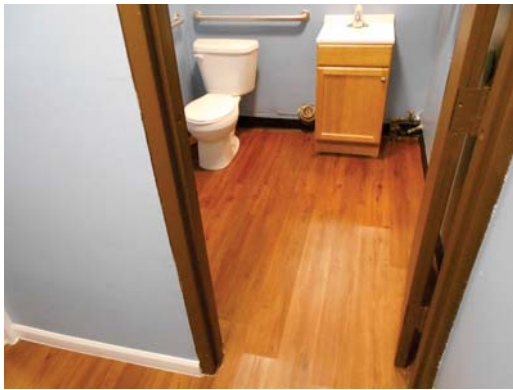
1801 Attucks, community building restroom
