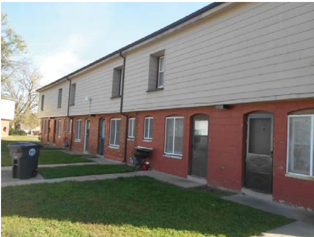
147. 921-935 Custer Place, rear facade
