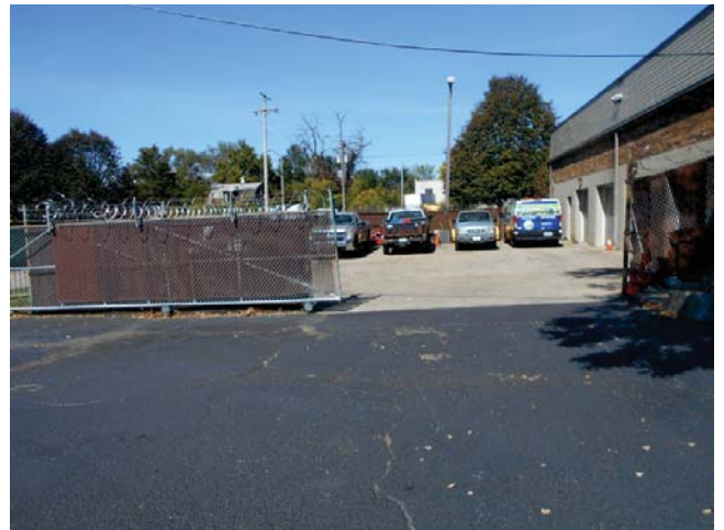
80. Leasing office asphalt parking lot
