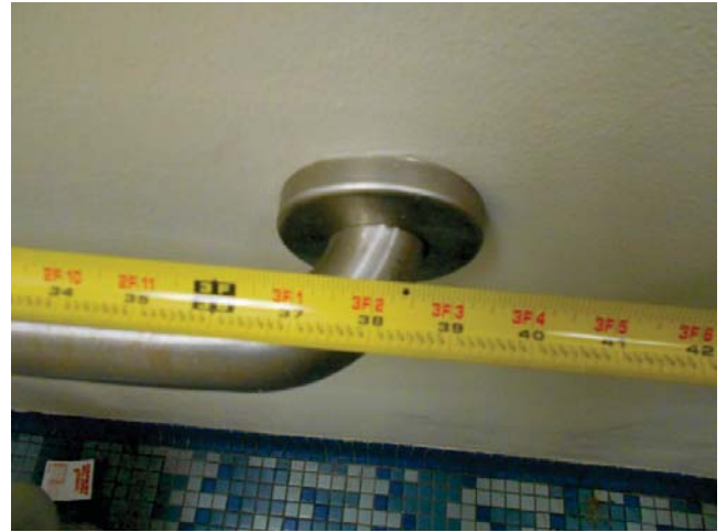
14. Leasing office public restroom, rear grab bar, 38"
