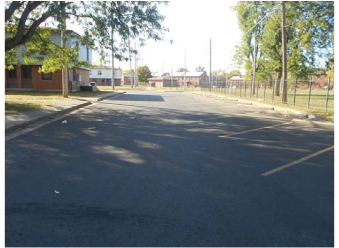
122. Newer asphalt pavement and seal coat
