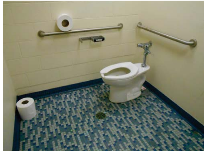
10. Leasing office public restroom
