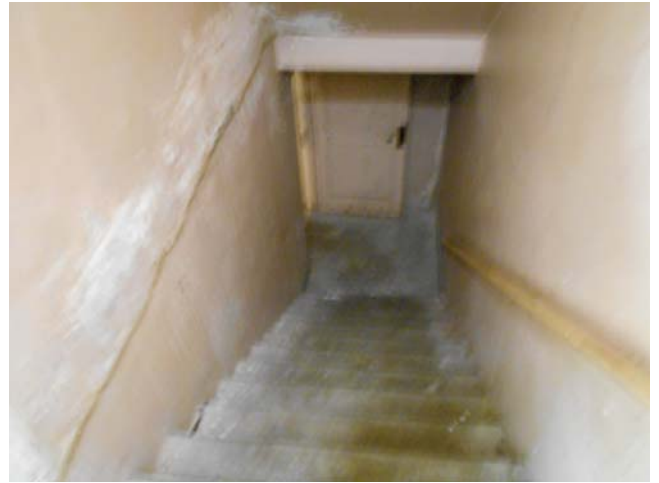
58. 900-914 Wilberforce Place, Task Force HQ, Mechanical Basement
