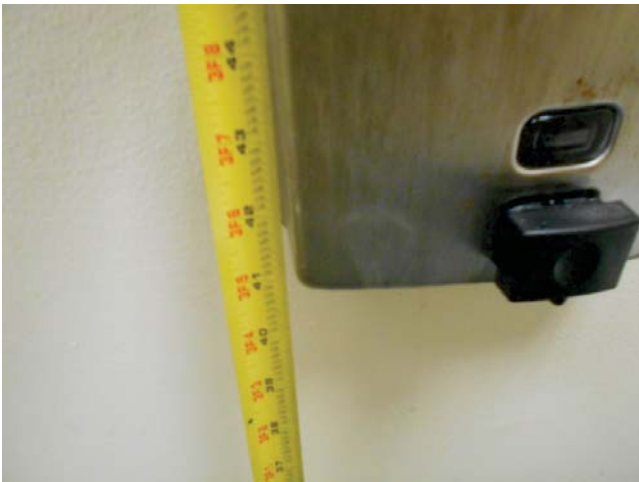
15. Leasing office public restroom, soap dispenser height, 41"
