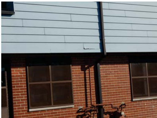
Typical section 502 building, older exterior siding
