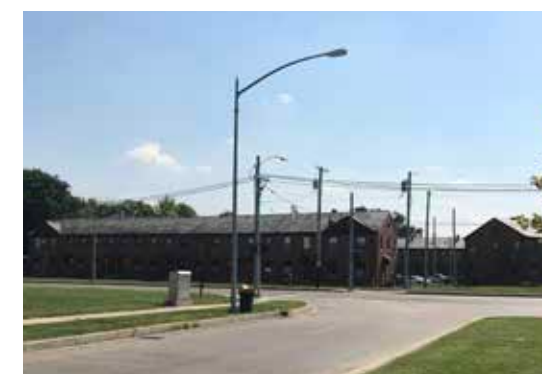
Existing conditions at DeSoto Bass
