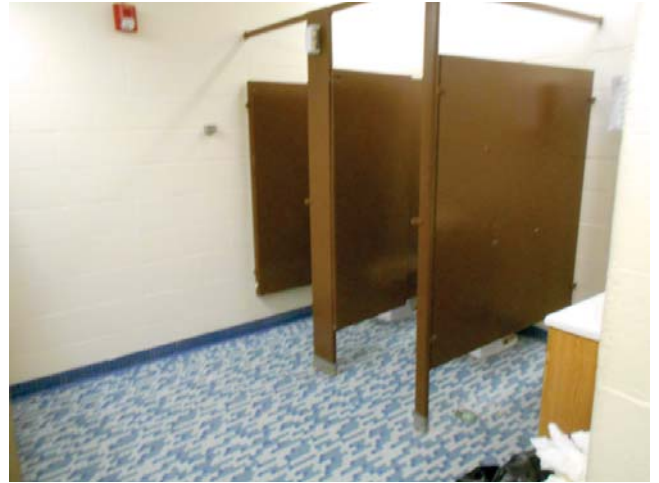
46. Leasing office maintenance offices restroom
