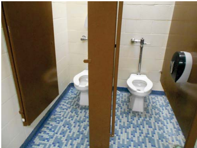
47. Leasing office maintenance offices restroom
