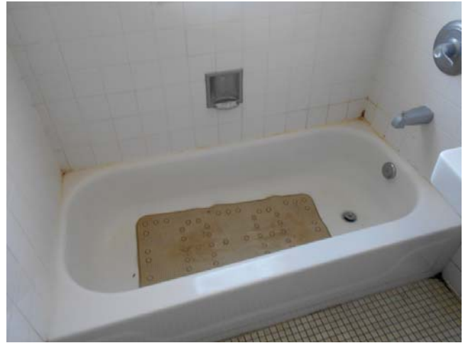
14. 818 Oldfield Avenue, 1bed/1bath, upstairs unit, vacant - Bathroom
