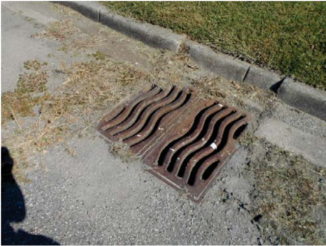
85. Paved area drainage
