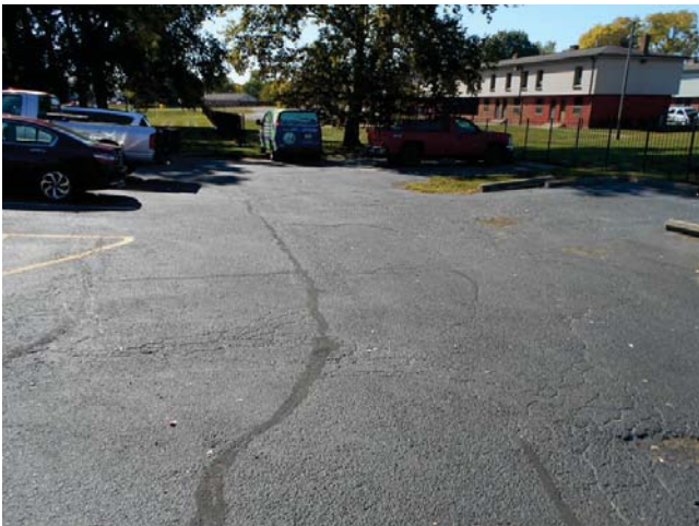
79. Leasing office asphalt parking lot
