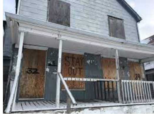
Figure 2 West Side Blight
