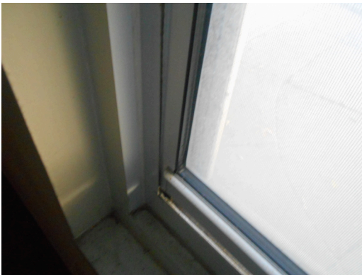
Unit E - 1bed/1bath, vacant - Vinyl windows
