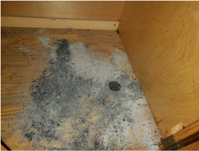
57. Update- Unit B - 1bed/1bath, vacant - 2nd Floor- Kitchen- Older Cabinet
