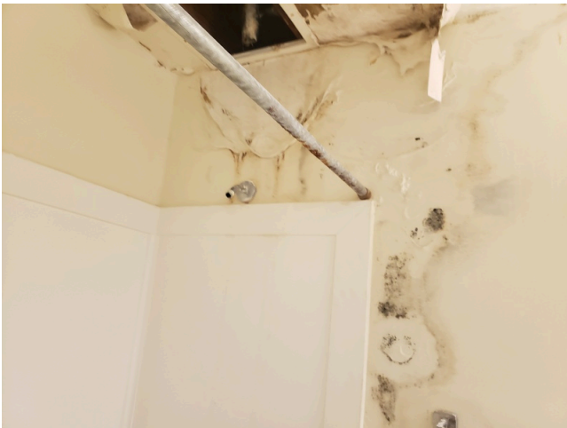
19. Update- Unit A - 1bed/1bath, vacant -Bedroom- Replace water wall
