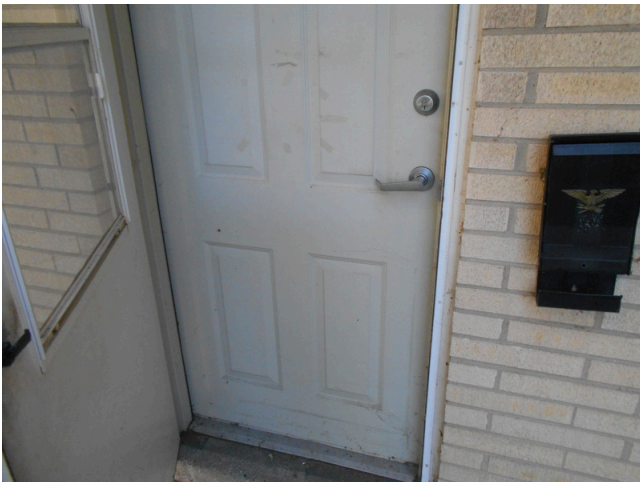
15. Typical exterior unit entrance door
