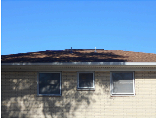
Asphalt shingle roofing
