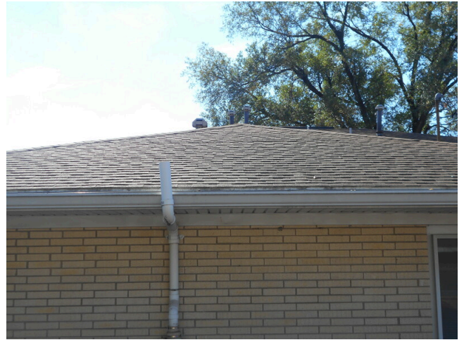
18. Asphalt shingle tile roofing
