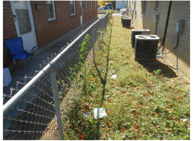
22. Chain link fencing
