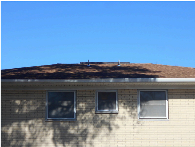
11. Asphalt shingle roofing
