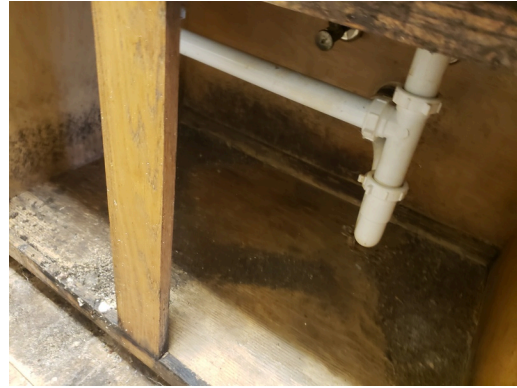
Update- Unit A - 1bed/1bath, vacant - Kitchen- Replace older cabinet
