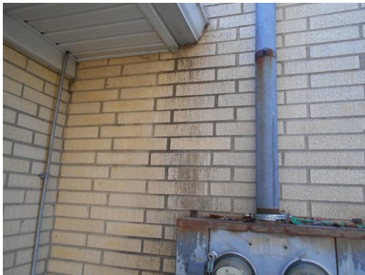
Cleaning of masonry
