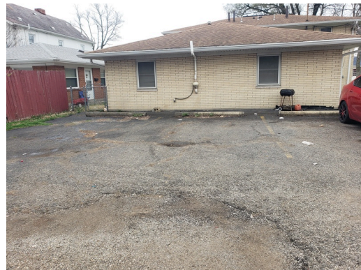
Asphalt shingle roofing
