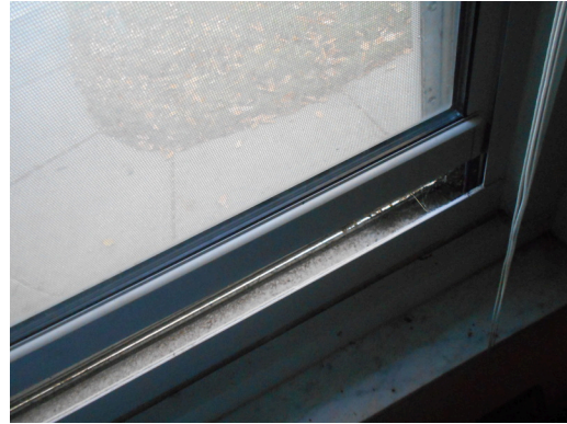
Unit E - 1bed/1bath, vacant - Vinyl windows
