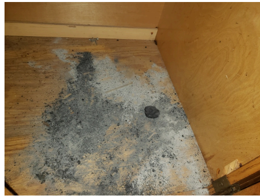
Update- Unit B - 1bed/1bath, vacant - 2nd Floor- Kitchen- Older Cabinet
