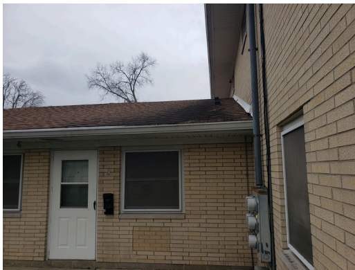
Cleaning of masonry
