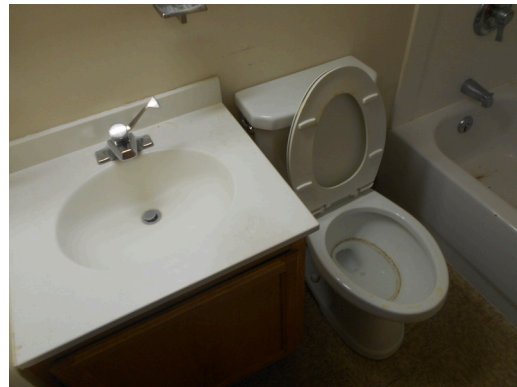
Unit E - 1bed/1bath, vacant - Bathroom
