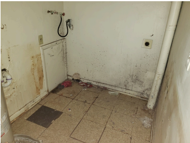
59. Update- Unit B - 1bed/1bath, vacant - 2nd Floor- Laundry Room- Damaged VCT flooring
