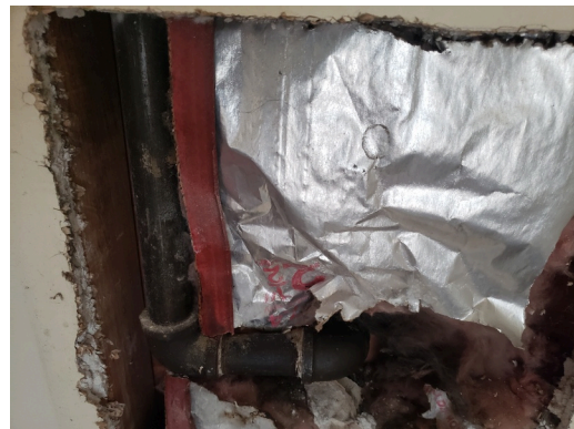
Update- Unit D - 1bed/1bath, vacant -Living Room- Plumbing
