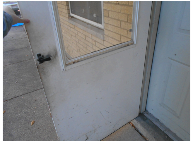
16. Typical exterior unit entrance screen door
