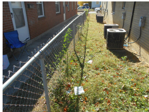
Chain link fencing
