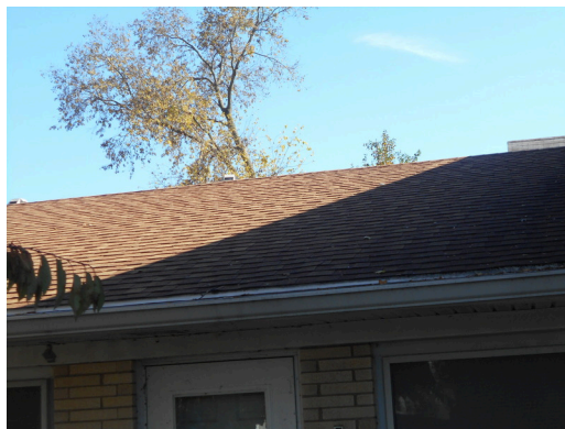
Asphalt shingle tiles
