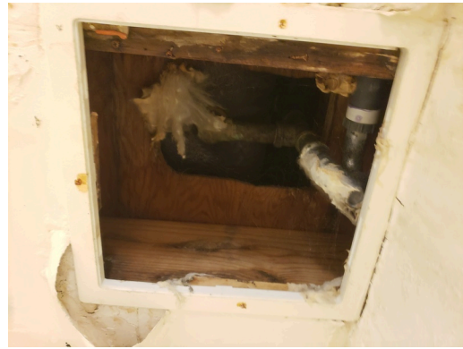
Update- Unit A - 1bed/1bath, vacant - Bathroom- Plumbing
