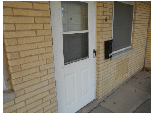
Typical exterior unit entrance door
