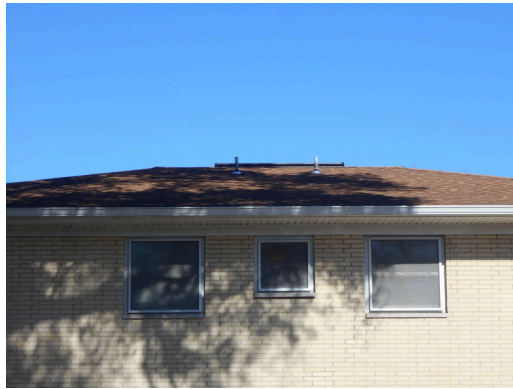
Asphalt shingle roofing
