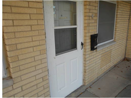
Typical exterior unit entrance door
