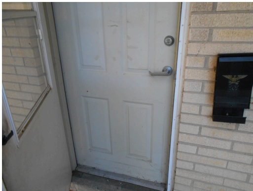
Typical exterior unit entrance door
