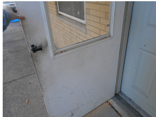
Typical exterior unit entrance screen door
