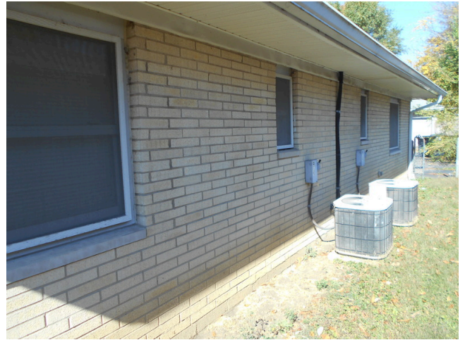
26. Site facade and old AC units
