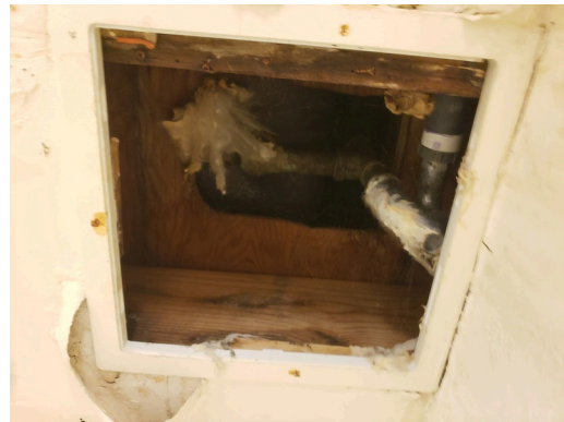
Update- Unit A - 1bed/1bath, vacant - Bathroom- Plumbing
