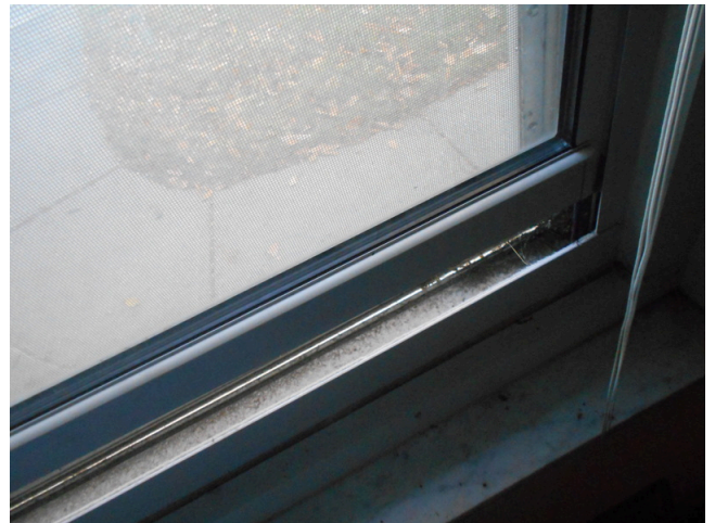
20. Unit E - 1bed/1bath, vacant - Vinyl windows
