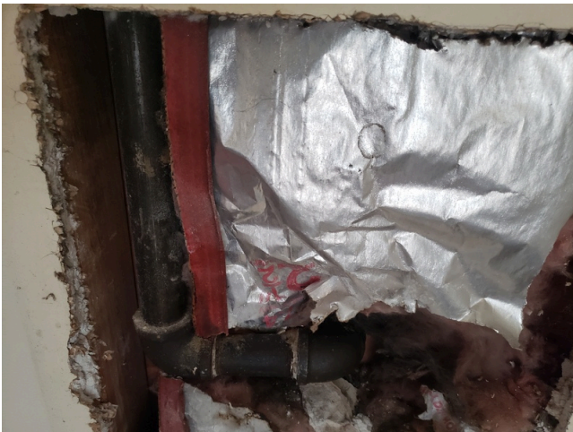
83. Update- Unit D - 1bed/1bath, vacant -Living Room- Plumbing
