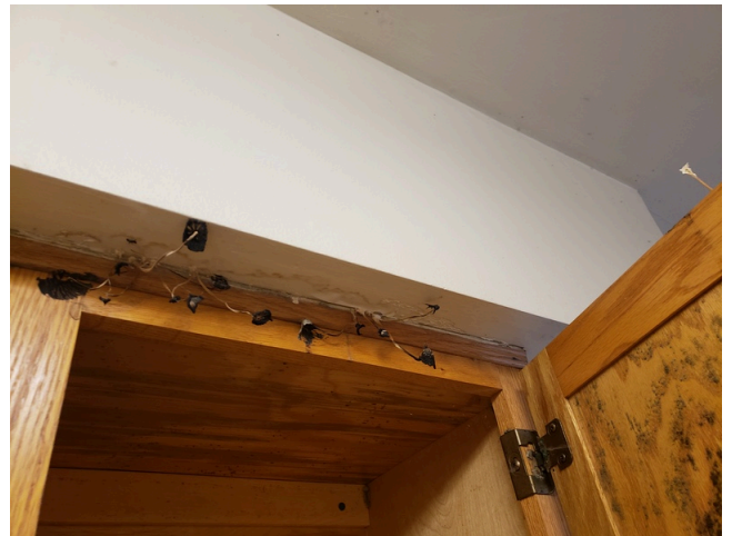
40. Update- Unit A - 1bed/1bath, vacant - Kitchen- Replace older cabinet
