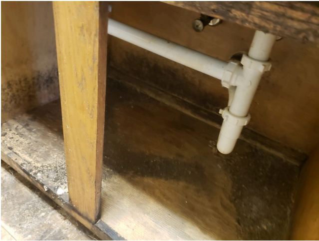
41. Update- Unit A - 1bed/1bath, vacant - Kitchen- Replace older cabinet
