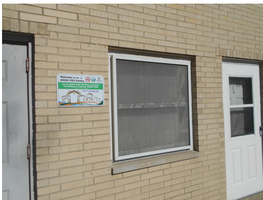
Cleaning of masonry
