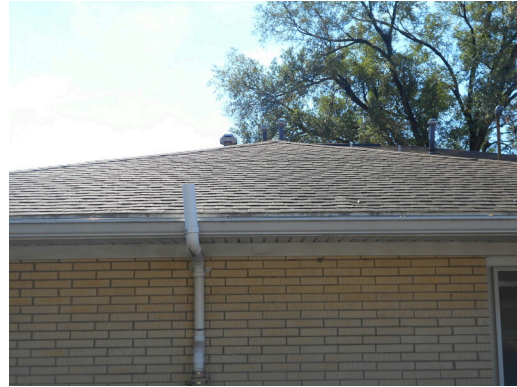
Asphalt shingle roofing
