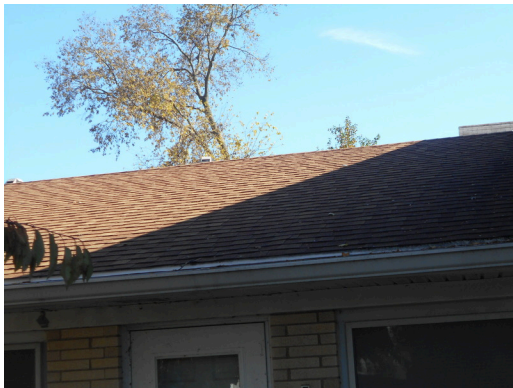
Asphalt shingle roofing
