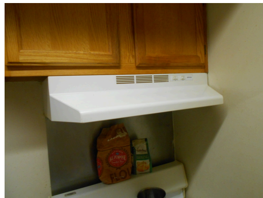
Unit F - 1bed/1bath - Kitchen range overhead shield
