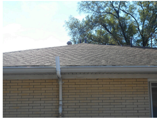
Asphalt shingle tile roofing
