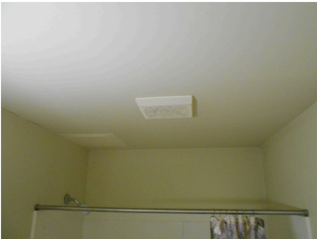
15. Unit D - 1bed/1bath, vacant - Bathroom ceiling
