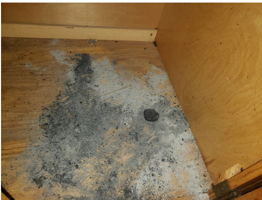
Update- Unit B - 1bed/1bath, vacant - 2nd Floor- Kitchen- Older Cabinet
