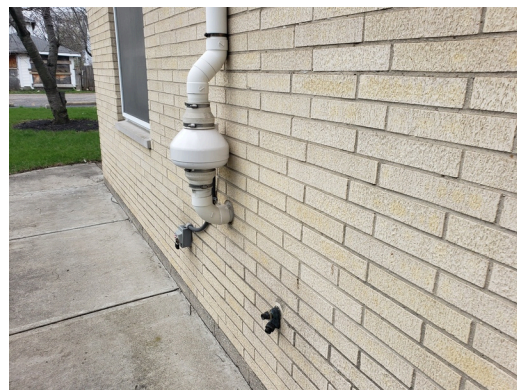
Cleaning of masonry
