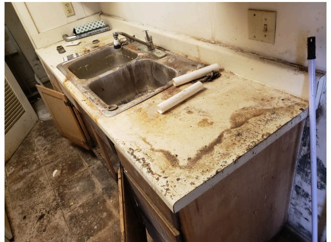
16. Update- Unit A - 1bed/1bath, vacant - Kitchen- Replace older cabinet
