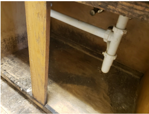
Update- Unit A - 1bed/1bath, vacant - Kitchen- Replace older cabinet
