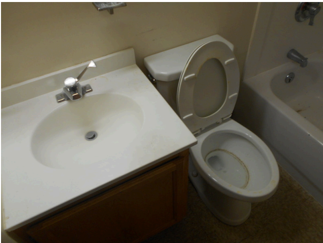
35. Unit E - 1bed/1bath, vacant - Bathroom
