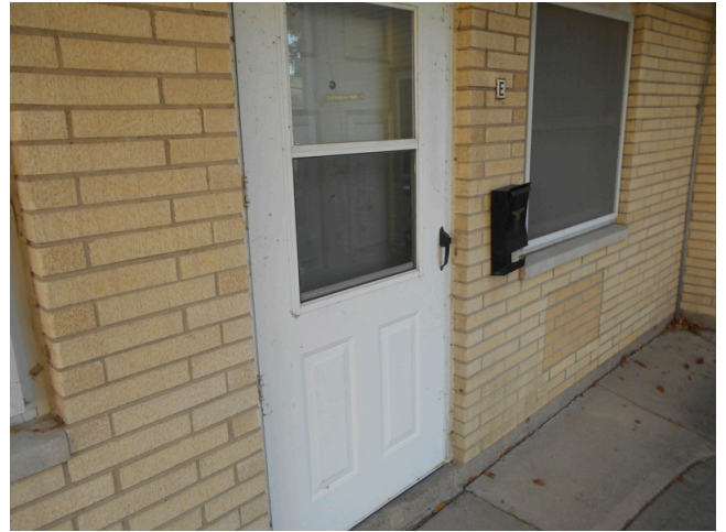
14. Typical exterior unit entrance door
