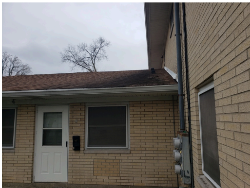
Asphalt shingle roofing
