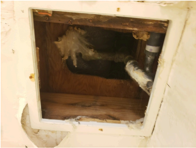
5. Update- Unit A - 1bed/1bath, vacant - Bathroom- Plumbing
