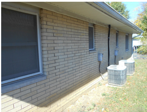
Site facade and old AC units
