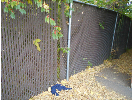
Chain link fencing
