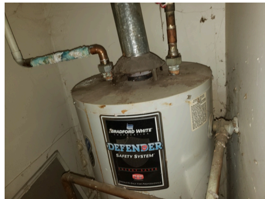
Unit 267-C - 1bed/1bath, occupied-(update)- 30-Gal water heater MFG-2003
