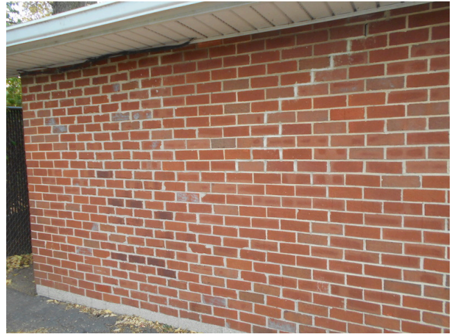
30. Typical brick facade
