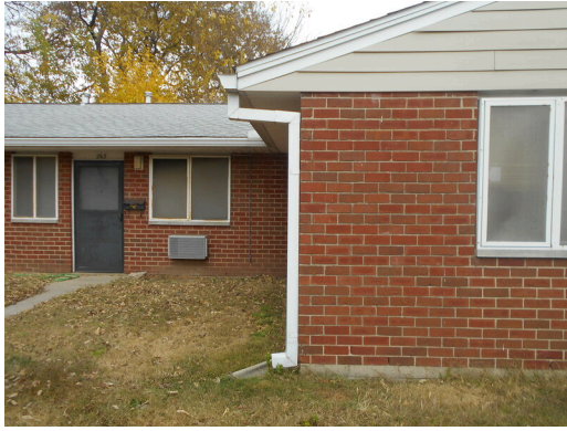
Gutter downspout
