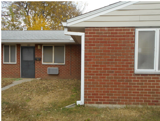
Gutter downspout
