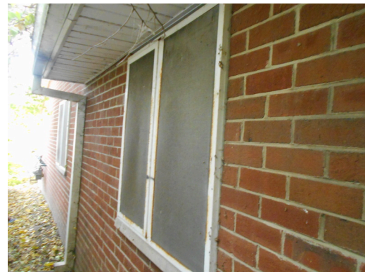
Typical window screens
