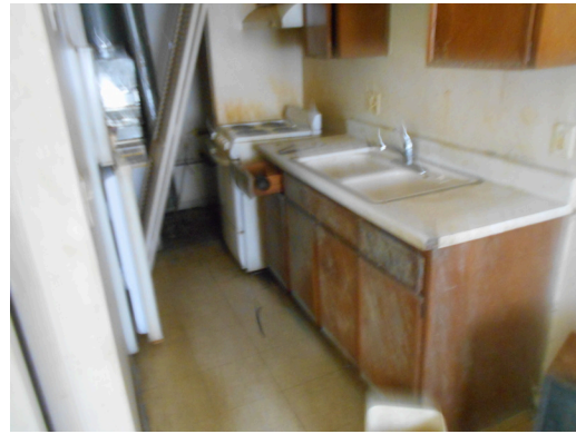
Unit 267-A - 1bed/1bath, vacant - Kitchen
