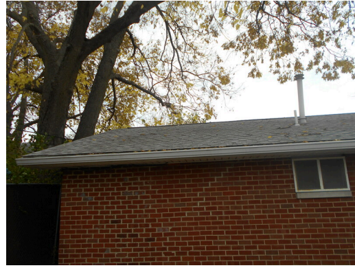
Asphalt shingle tile roofing
