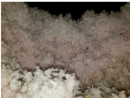
Blown-in insulation
