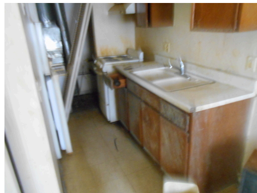
Unit 267-A - 1bed/1bath, vacant - Kitchen
