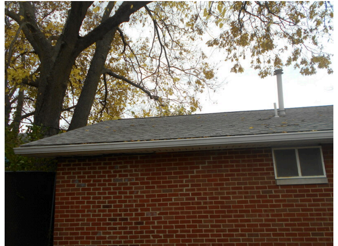
4. Asphalt shingle tile roofing
