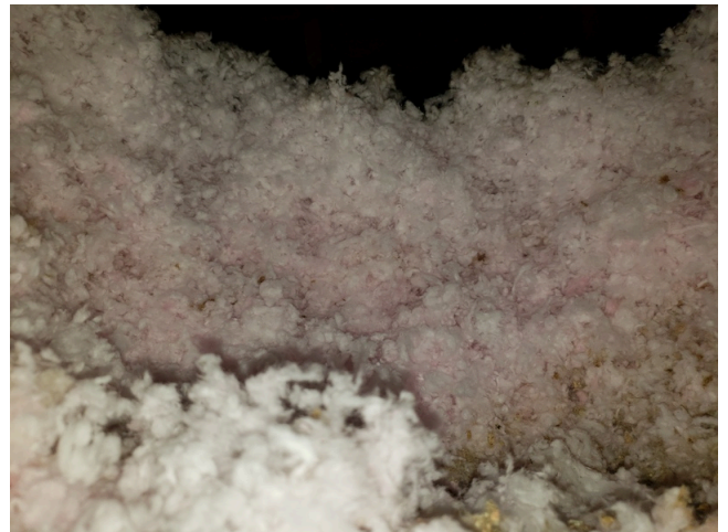
32. Blown-in insulation
