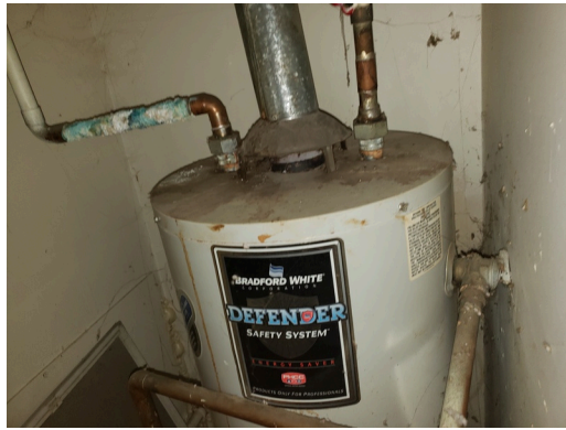
Unit 267-C - 1bed/1bath, occupied-(update)- 30-Gal water heater MFG-2003
