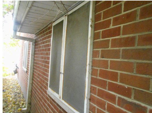
Typical window screens
