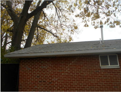
Asphalt shingle tile roofing
