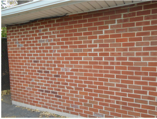
Typical brick facade
