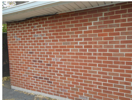
Typical brick facade
