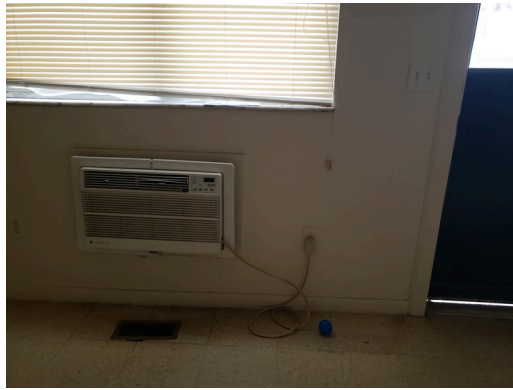
Unit 265- D - 1bed/1bath,vacant-(update)- Through wall ac unit
