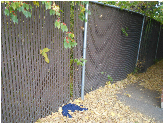
5. Chain link fencing
