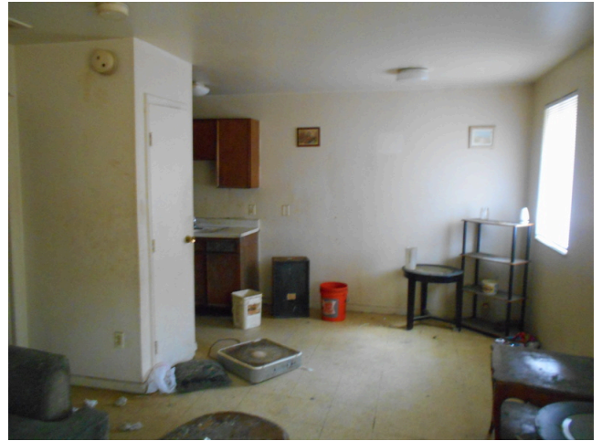
50. Unit 267-A - 1bed/1bath, vacant - Living area
