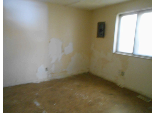
Unit 261 - 1bed/1bath, vacant - Bedroom
