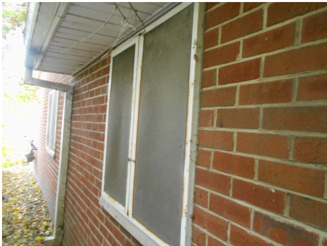
11. Typical window screens
