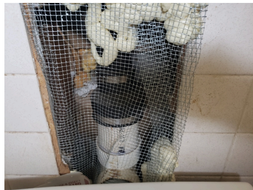
Unit 267-C - 1bed/1bath, occupied-(update)- Bathroom- Damaged tile
