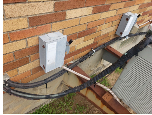
Update- HVAC Units replace insulation
