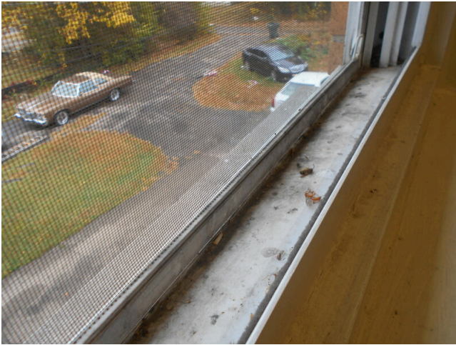
17. Common area stairwell window
