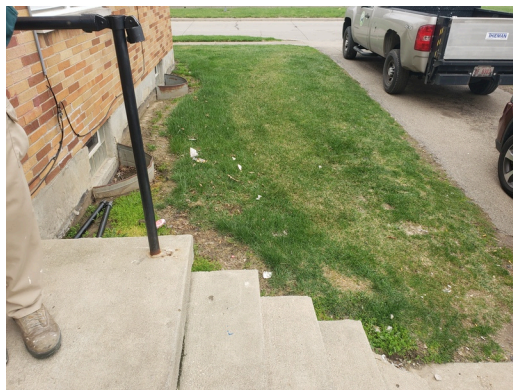
Update- Main entry stair- repair damaged stair railing
