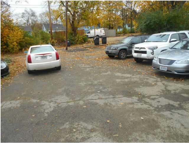
49. Asphalt parking lot
