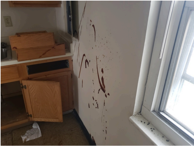
25. Update- Unit A, 2 bedroom/1 bathroom- Kitchen- Paint
