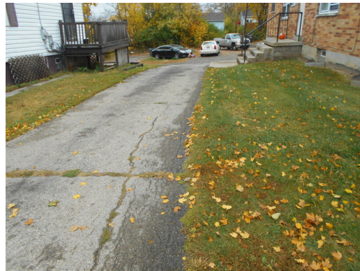
Site entrance from North Gettysburg Avenue
