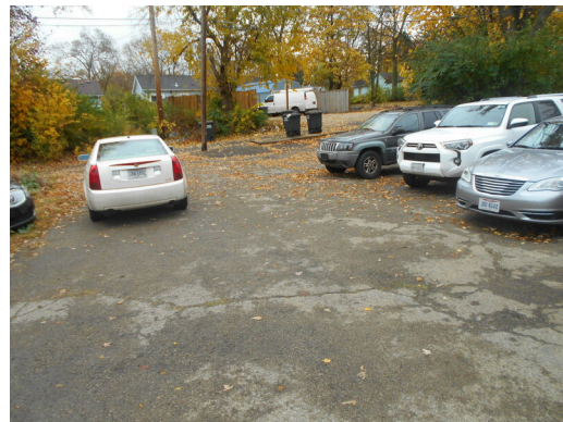
Asphalt parking lot
