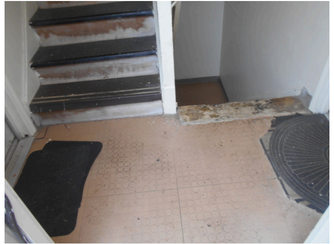
46. Common area stairwell entrance
