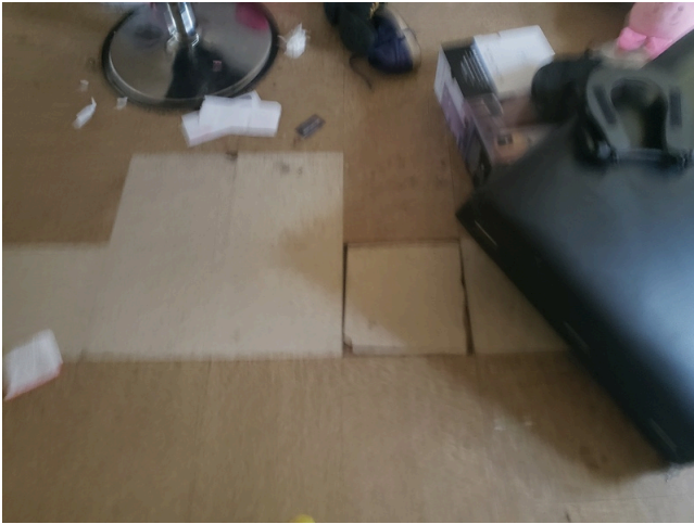
45. Update- Unit C, 2 bedroom/1 bathroom- Living room- damaged VCT
