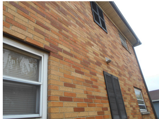
Typical brick facade
