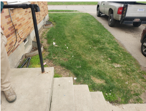
Update- Main entry stair- repair damaged stair railing
