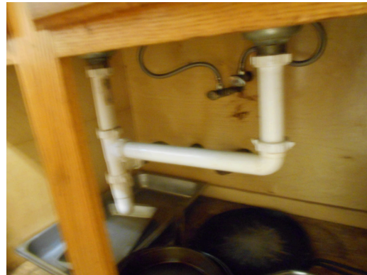
Unit E, 2 bedroom/1 bathroom - Kitchen sink
