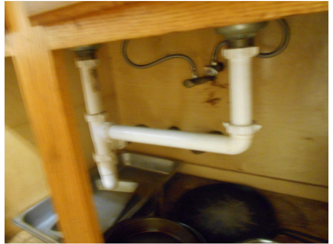
14. Unit E, 2 bedroom/1 bathroom - Kitchen sink
