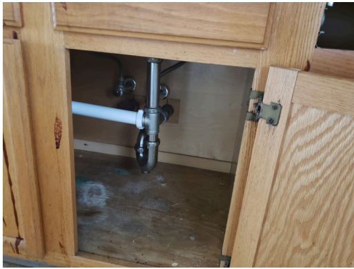
Update- Unit A, 2 bedroom/1 bathroom- kitchen- Plumbing
