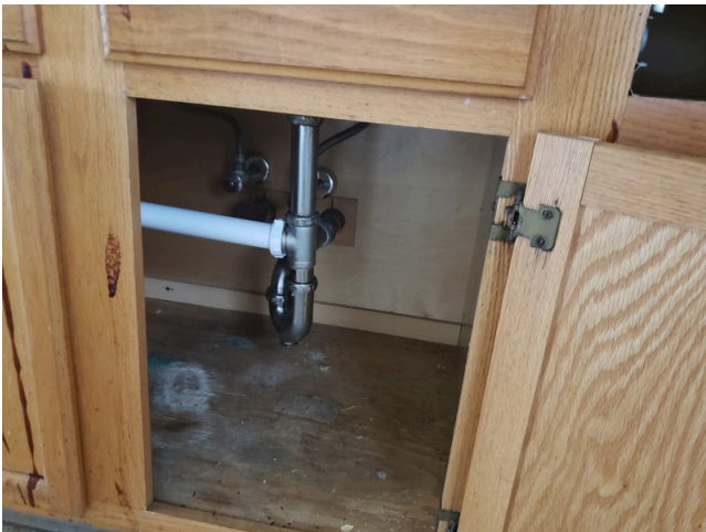
23. Update- Unit A, 2 bedroom/1 bathroom- kitchen- Plumbing
