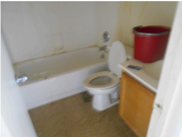
47. Unit A, 2 bedroom/1 bathroom, vacant - Bathroom
