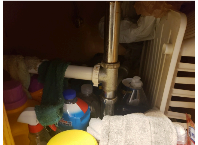
18. Update- Unit D, 2 bedroom/1 bathroom- Kitchen- Plumbing
