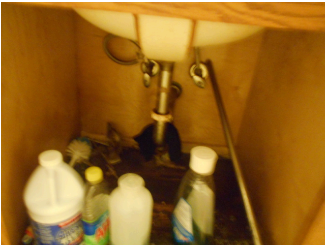
19. Unit E, 2 bedroom/1 bathroom - Bathroom sink
