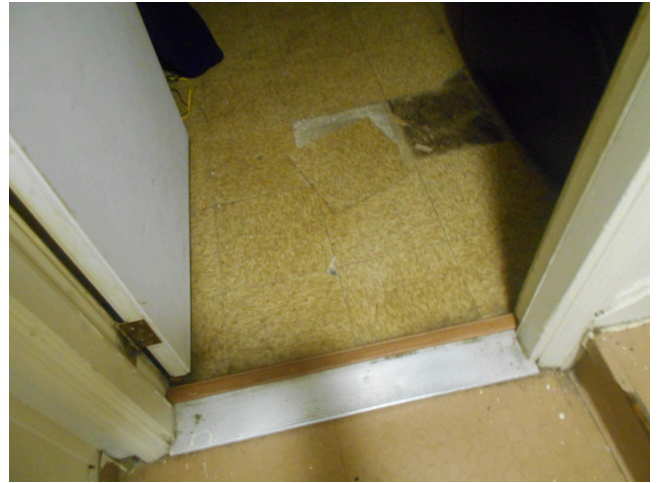
2. Unit E, 2 bedroom/1 bathroom - Threshold
