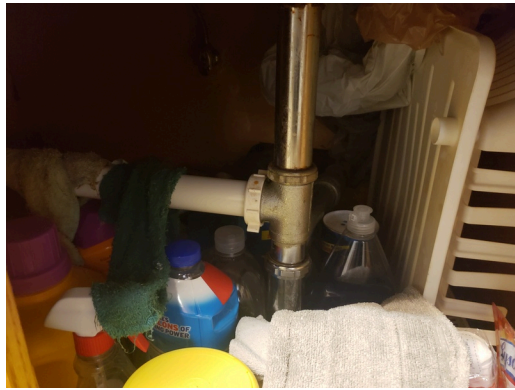
Update- Unit D, 2 bedroom/1 bathroom- Kitchen- Plumbing
