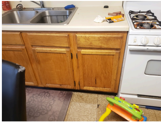
Update- Unit C, 2 bedroom/1 bathroom- Kitchen Cabinet
