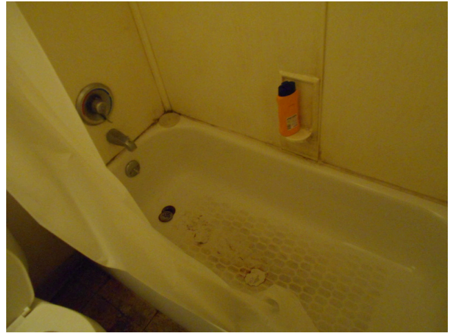
22. Unit E, 2 bedroom/1 bathroom - Bathroom shower
