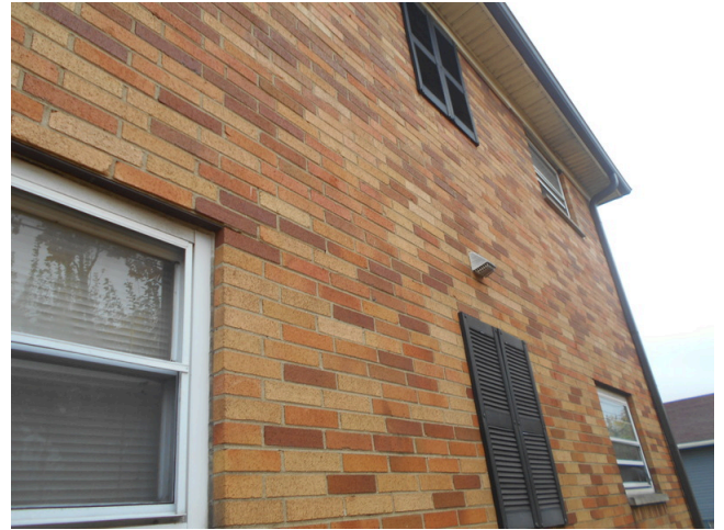
26. Typical brick facade
