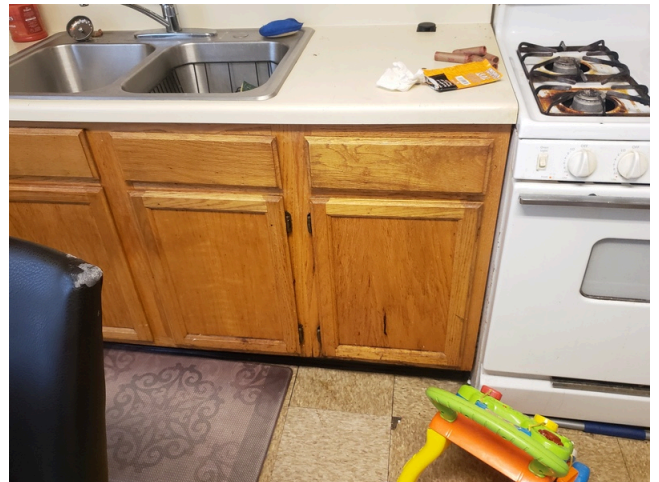
52. Update- Unit C, 2 bedroom/1 bathroom- Kitchen Cabinet
