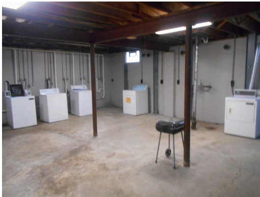
Common area laundry room
