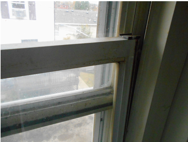
31. Unit A, 2 bedroom/1 bathroom, vacant - Vinyl window
