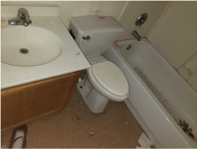
5. Update- Unit C, 2 bedroom/1 bathroom- Bathroom
