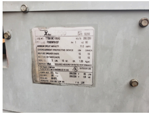
Update- HVAC 1.5 Ton- MFR- 2002
