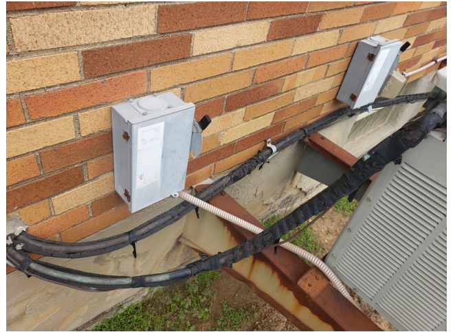
34. Update- HVAC Units replace insulation
