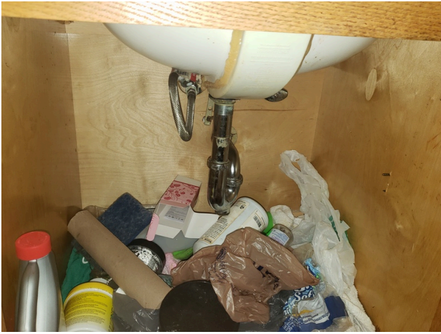
37. Update- Unit C, 2 bedroom/1 bathroom- Bathroom- Vanity
