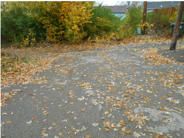
51. Asphalt parking lot
