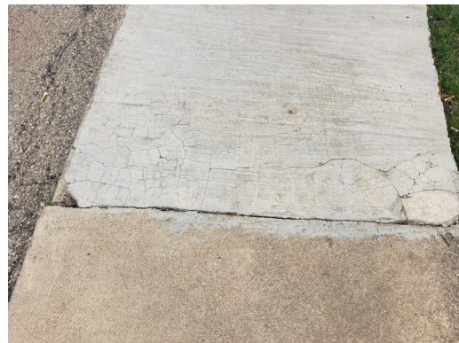
Update- Repair cracking concrete sidewalk
