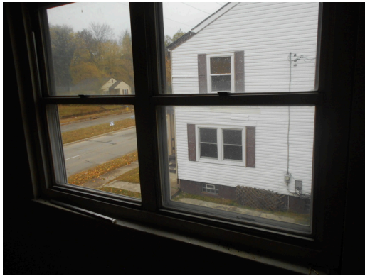
Unit A, 2 bedroom/1 bathroom, vacant - Vinyl window
