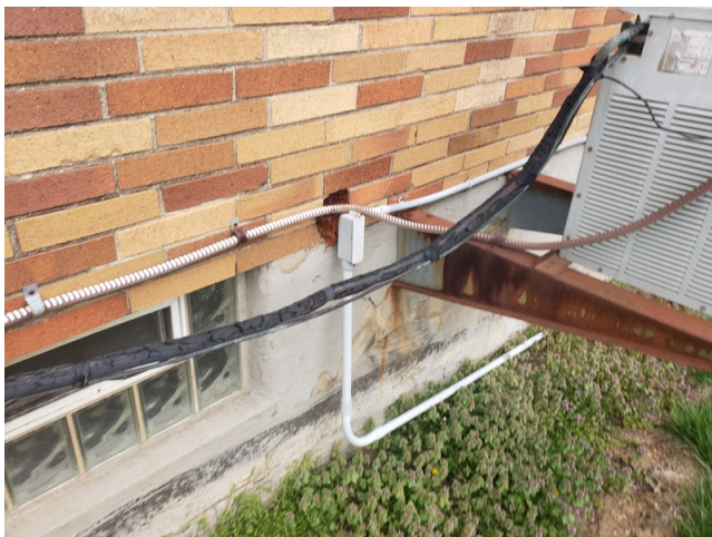
7. Update- HVAC Units replace insulation
