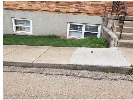
Update- Main sidewalk- install railings and rest area in ramp
