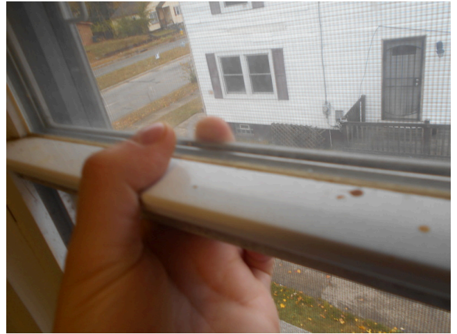
18. Common area stairwell window, double pane
