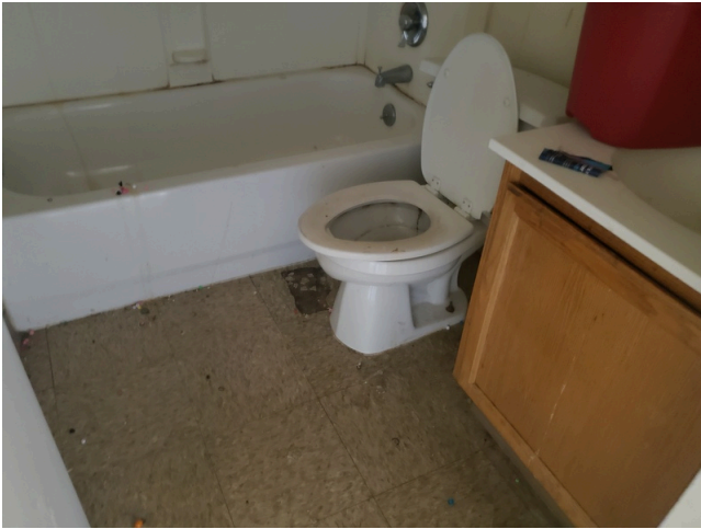
17. Update- Unit A, 2 bedroom/1 bathroom- Bathroom- repair damage VCT
