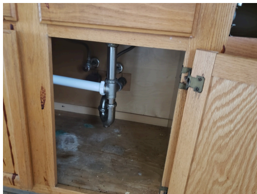
Update- Unit A, 2 bedroom/1 bathroom- kitchen- Plumbing
