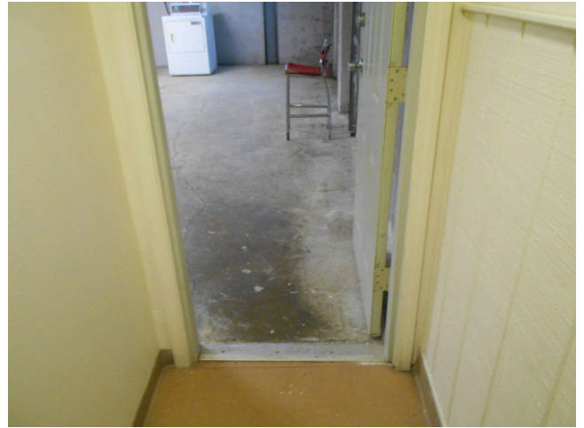
2. Entrance to basement common area laundry room
