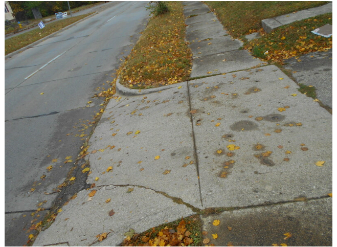
22. Site entrance from North Gettysburg Avenue
