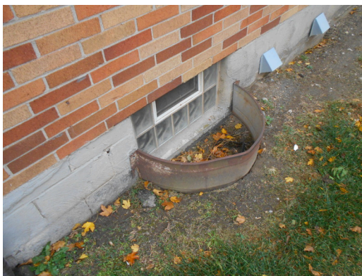
Brick veneer at window well
