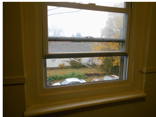
Common area stairwell window
