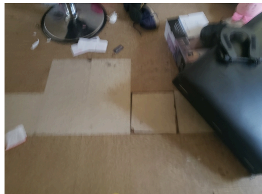
Update- Unit C, 2 bedroom/1 bathroom- Living room- damaged VCT
