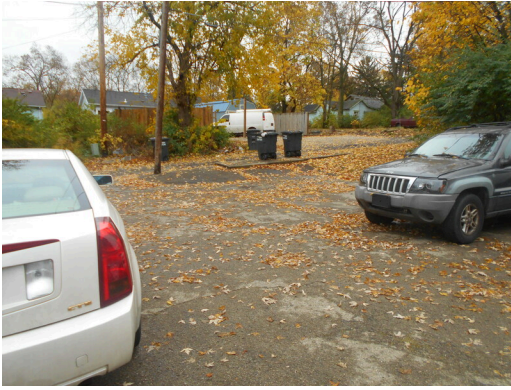
Asphalt parking lot
