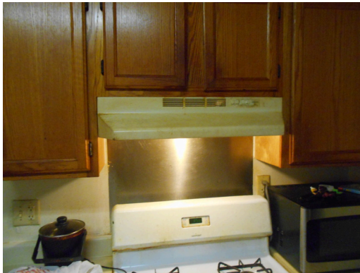
Unit E, 2 bedroom/1 bathroom - Kitchen overhead
