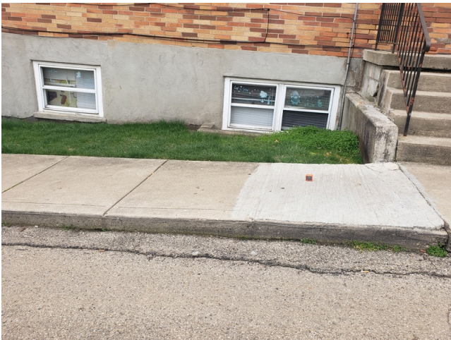
19. Update- Main sidewalk- install railings and rest area in ramp
