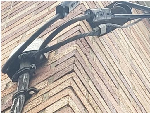
Electrical weatherhead
