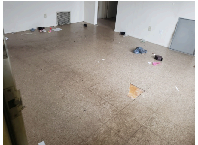
22. Update- Unit A, 2 bedroom/1 bathroom- Living room- repair damaged VCT
