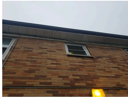
Soffit and fascia
