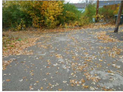
Asphalt parking lot
