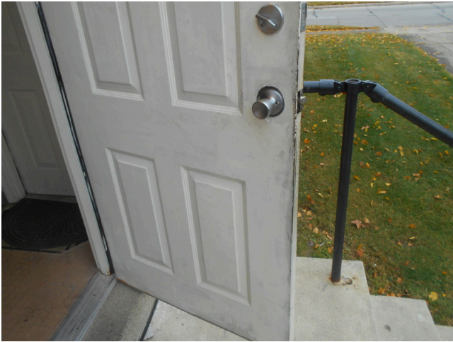
45. Building entrance door
