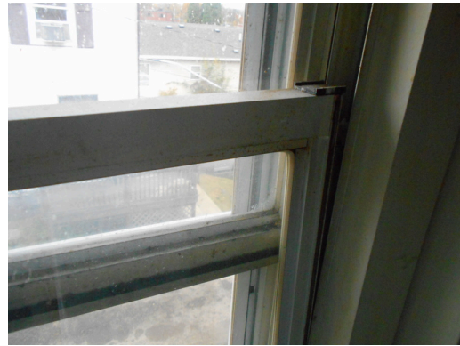
Unit A, 2 bedroom/1 bathroom, vacant - Vinyl window
