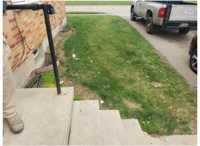
30. Update- Main entry stair- repair damaged stair railing
