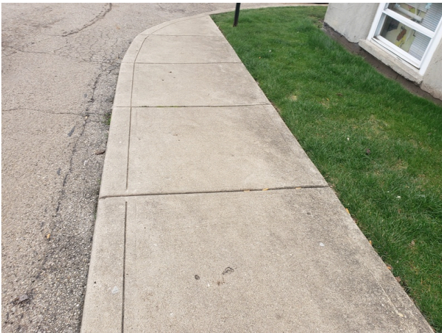
15. Update- Main sidewalk- install railings and rest area in ramp
