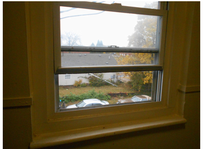
16. Common area stairwell window
