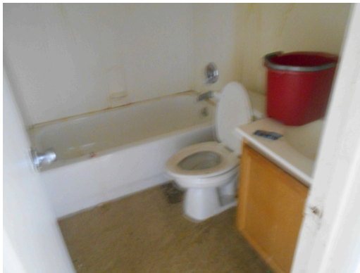
Unit A, 2 bedroom/1 bathroom, vacant - Bathroom
