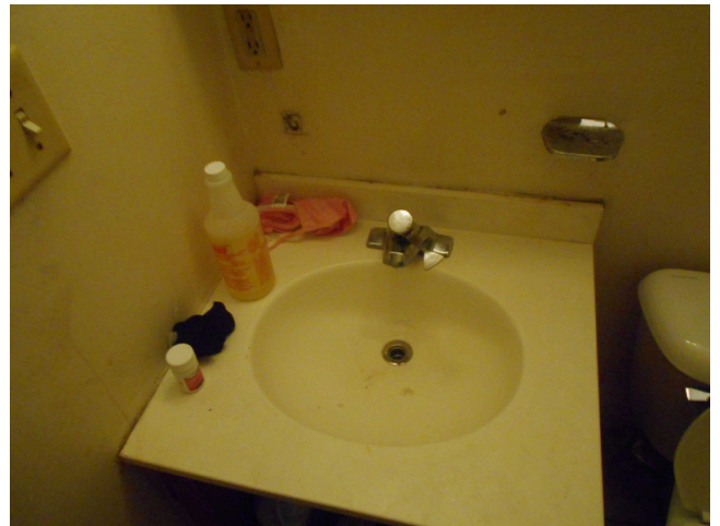
20. Unit E, 2 bedroom/1 bathroom - Bathroom sink
