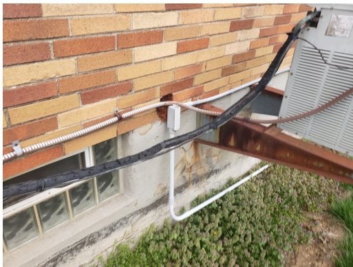
Update- HVAC Units replace insulation
