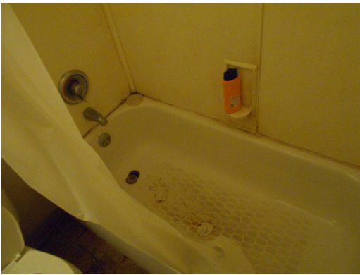
Unit E, 2 bedroom/1 bathroom - Bathroom shower
