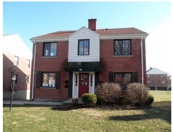
Pictured above is 538 Telford. While this property is owned by GDPM, it is not part of the Telford-Shroyer RAD Conversion. The building is located within 250 feet from 514 Telford. The 514 households will temporarily relocate to the 538 Telford building. Because of its proximity to the Telford-Shroyer units and because it's substantially similar in design, the relocation to 538 Telford should minimize the impact of the temporary displacement of the Telford-Shroyer households.
